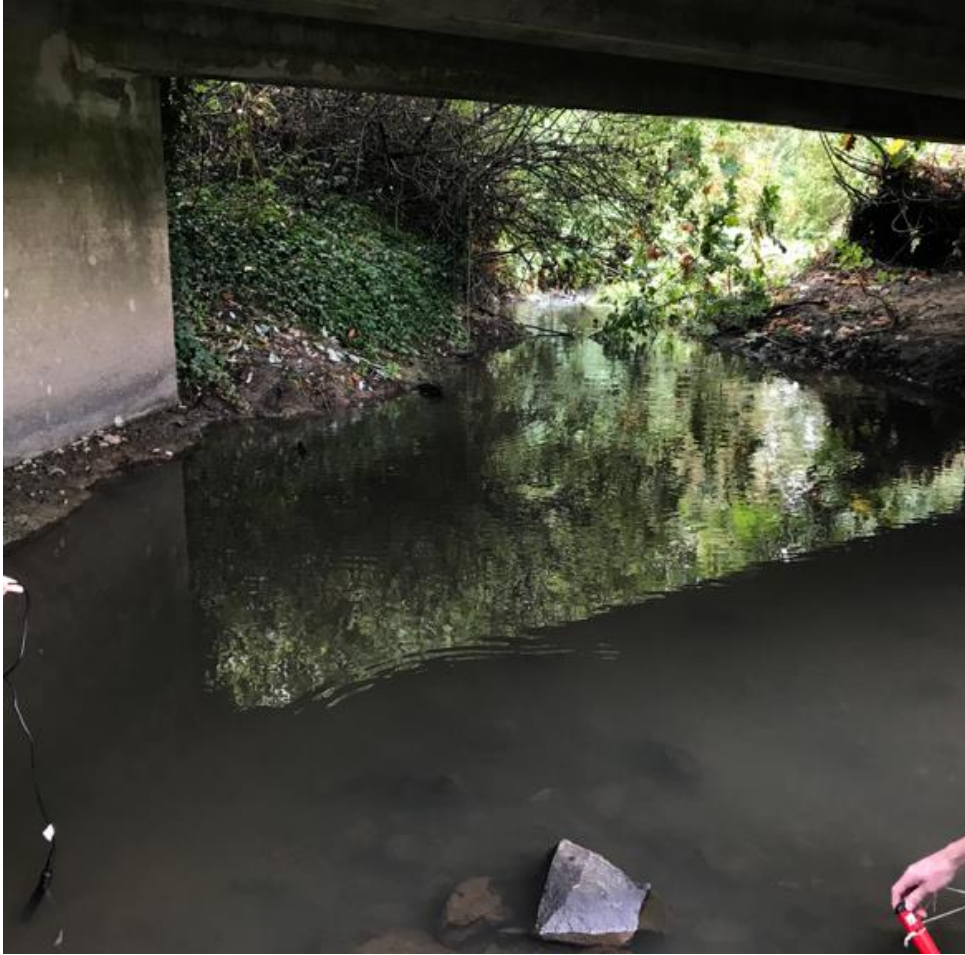
Image 2. Cozine Creek as viewed looking upstream under the Old Sheridan Bridge at site three. Photo taken 2017 by Kyle Huizinga
