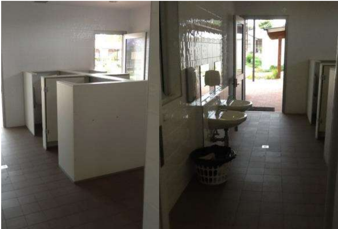
Figures 108 A & B: Taikurrendi Children and Family Centre – Children's Toilets
