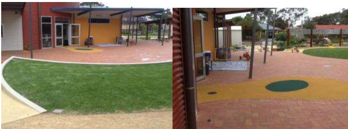
Figures 110 A & B: Taikurrendi Children and Family Centre – Entrance to Preschool & Grassed Area
