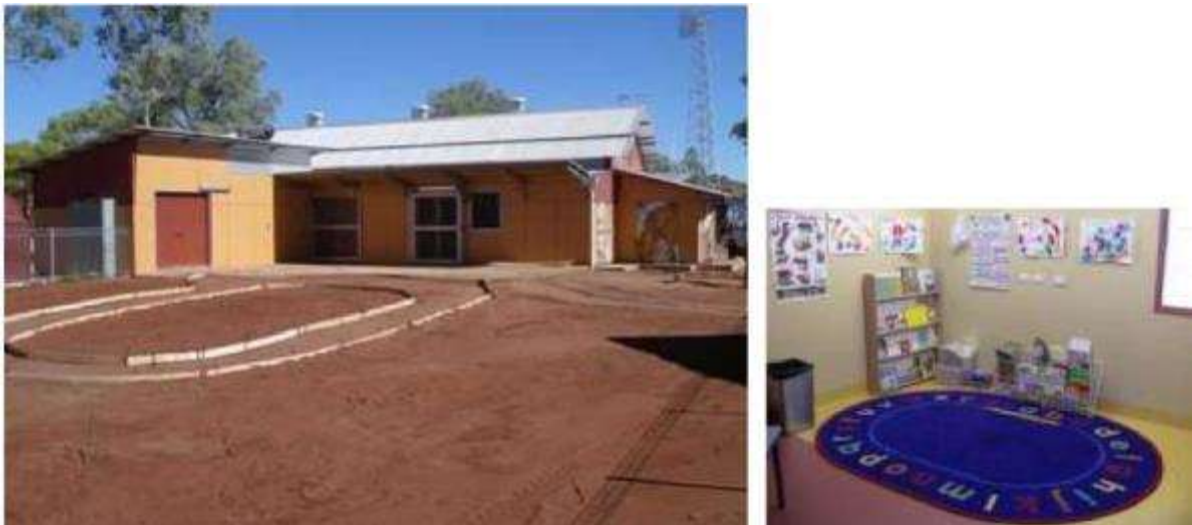
Figure 68: Pukatja (Ernabella) Children and Family Centre - External and internal outlooks (Source: Grant 2011).
