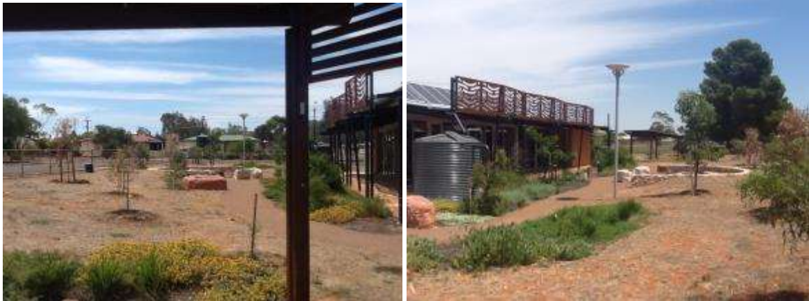
Figures 151 A & B: Gabmididi Manoo Children and Family Centre – Garden The planting in the garden on the western side of the centre has been lost due to poor maintenance.
