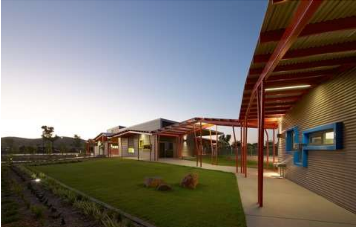
Figure 38: Roebourne Children and Family Centre - External areas between buildings (Source: Finn Pederson, 2014).
