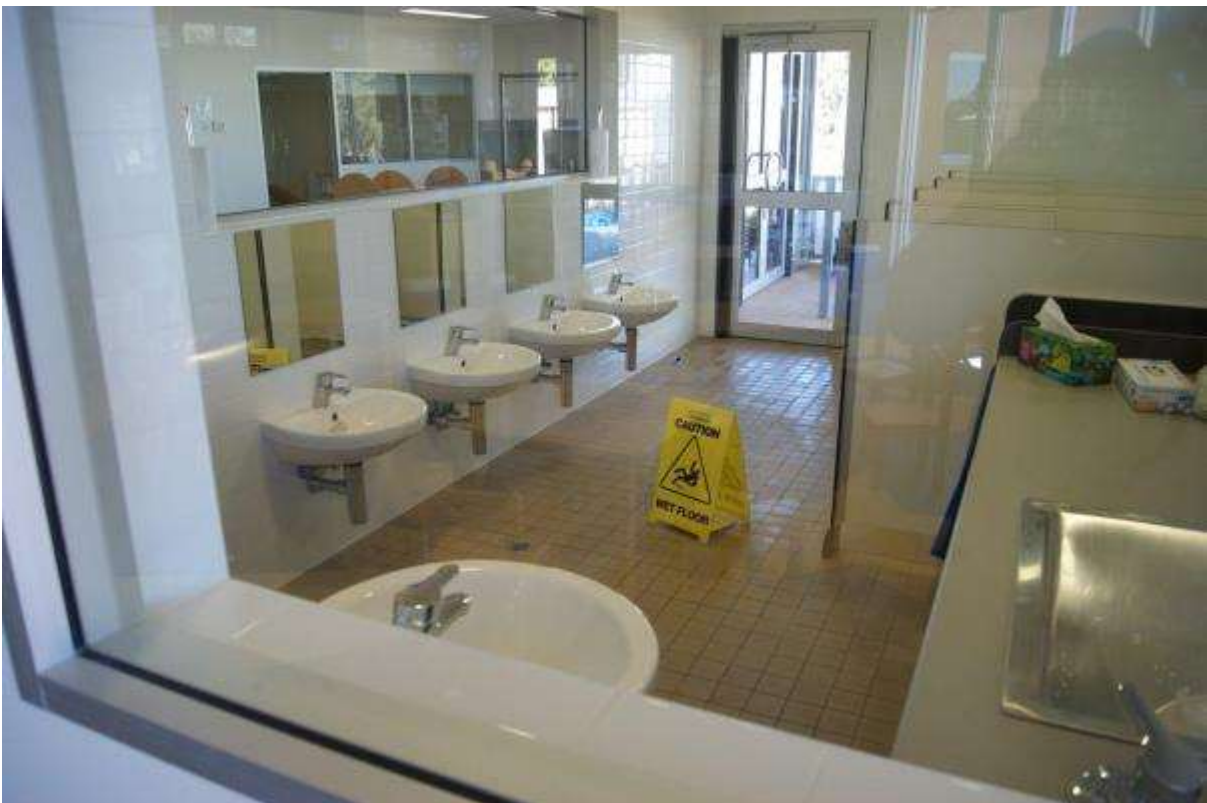
Figure 183: Ceduna Children and Family Centre - Preschool/Occasional Care Toilets
