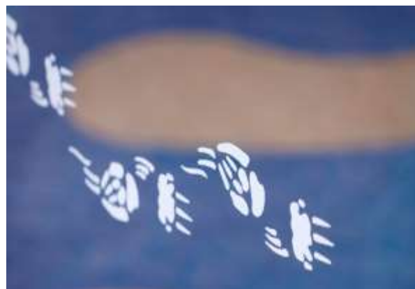
Figure 79: Taikurrendi Children and Family Centre – Etchings on Windows. Echidna paw prints are printed on the full length windows to both deter people from walking into them and repeat of the Kurna motif.
