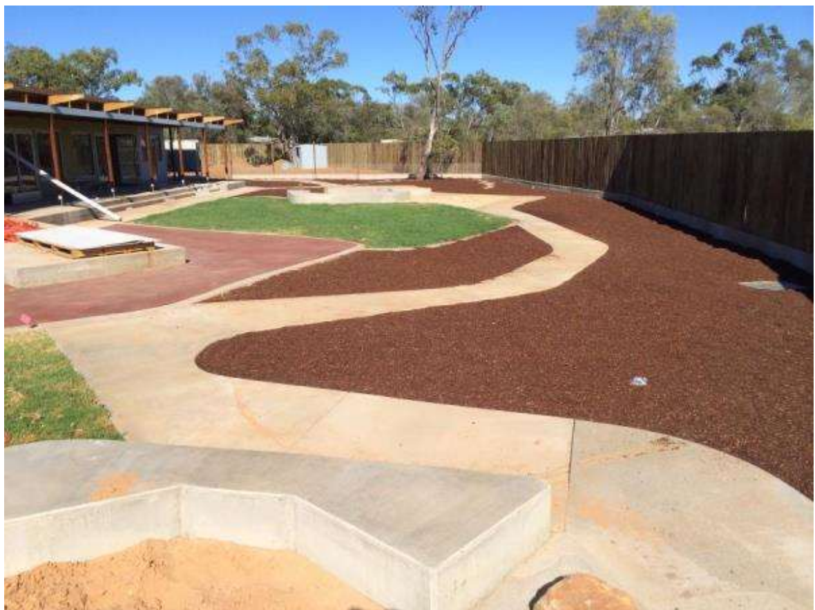
Figure 17: Lightning Ridge Aboriginal Integrated Child and Family Centre – Exterior.
