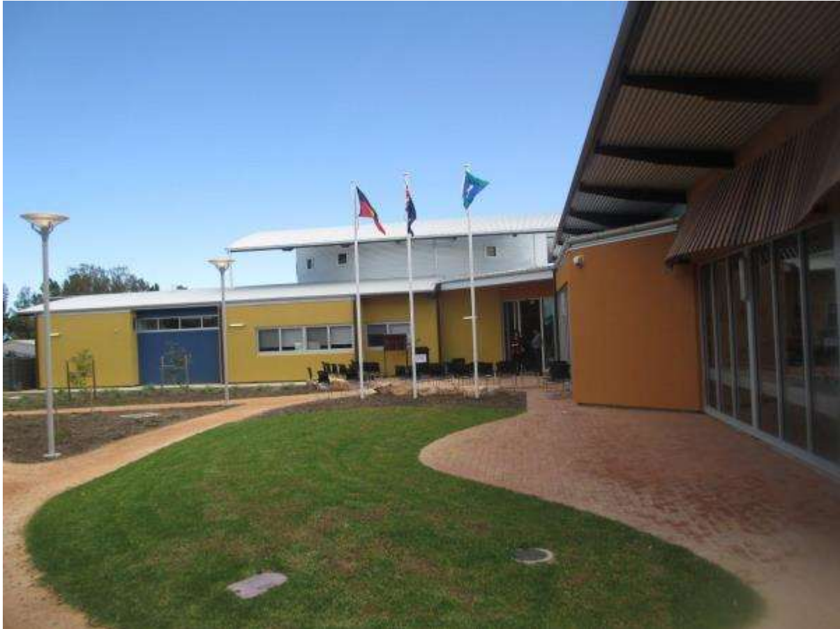
Figure 177: Ngura Yadurirn Children and Family Centre – Main Entrance
