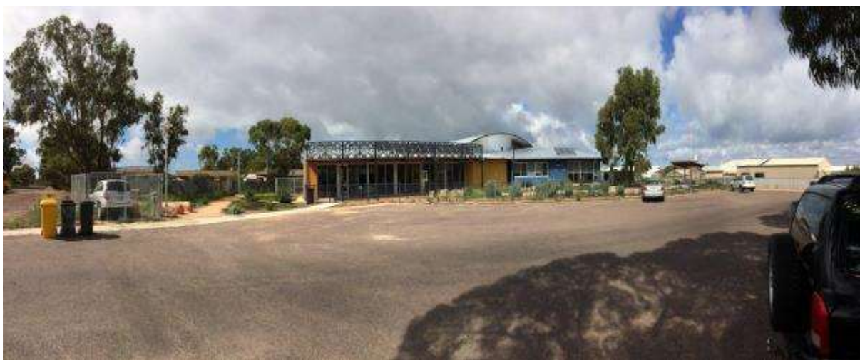
Figure 163: Ngura Yadurirn Children and Family Centre - Entrance from the Ceduna Area School car park
