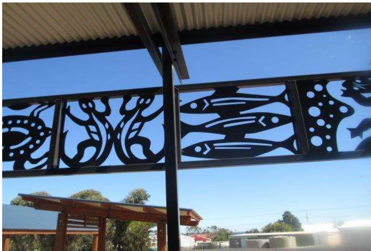
Figure 167: Ngura Yadurirn Children and Family Centre – Detail of lattice work
