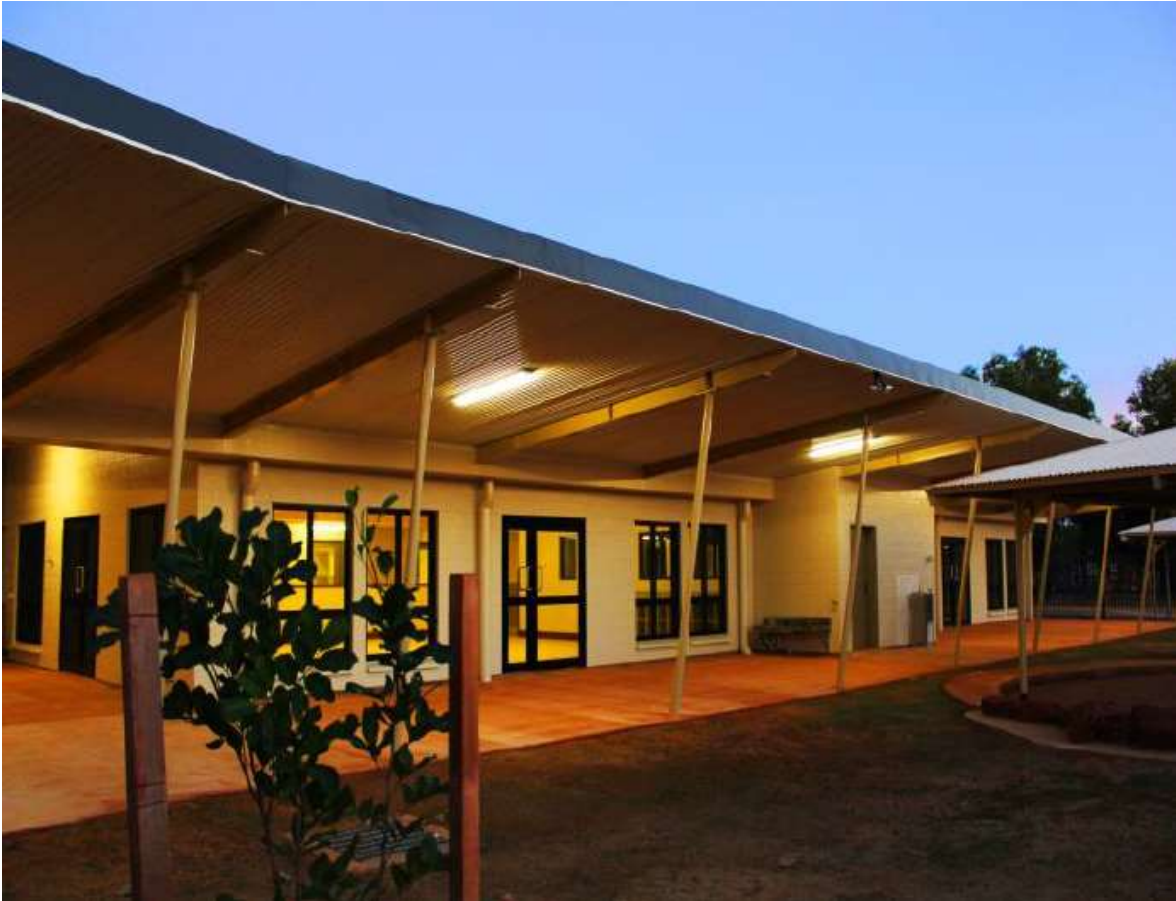
Figure 57: Ngukkurr Children and Family Centre – Exterior (Source: Ri-con 2014).
