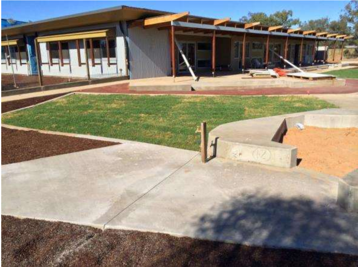
Figure 16: Lightning Ridge Aboriginal Integrated Child and Family Centre – Exterior.
