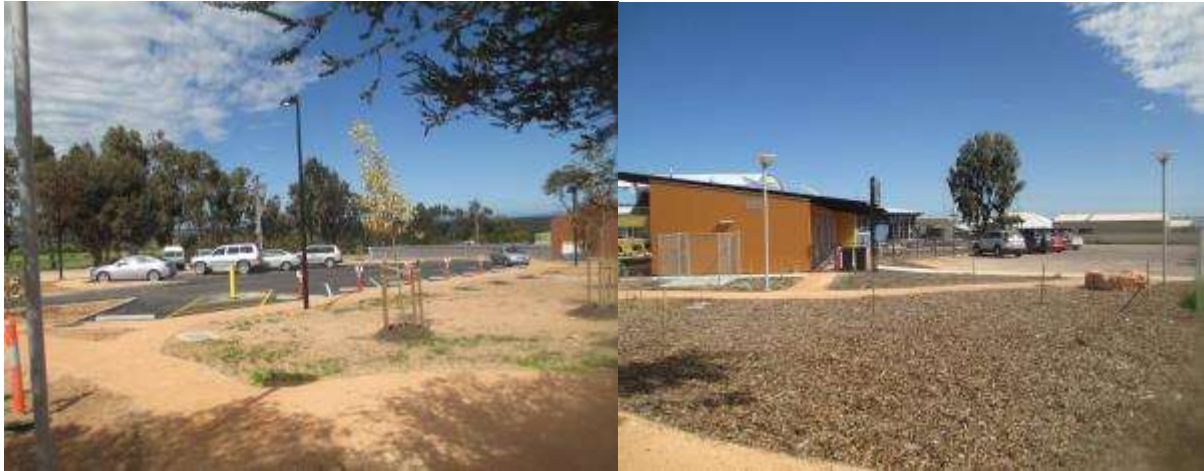
Figures: 176 A & B Ngura Yadurirn Children and Family Centre – Views of southern car park and eastern Ceduna Area School car park.
