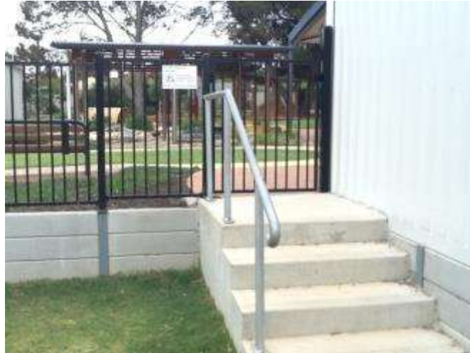
Figure 88: Taikurrendi Children and Family Centre - Connecting Gate from Primary School.
