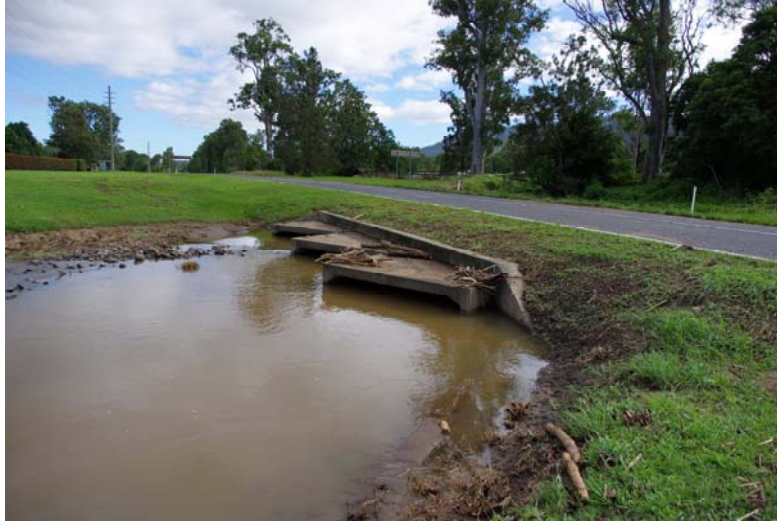
(a) Culvert outlet beneath Canungra-Tamborine Road QLD (Australia) on 31 March 2017
