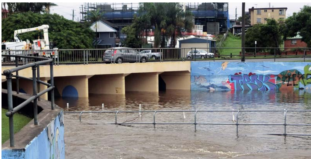
(c) Culvert inlet in operation on Norman Creek, Brisbane (Australia) on 25 February 2018 for a relatively small discharge
