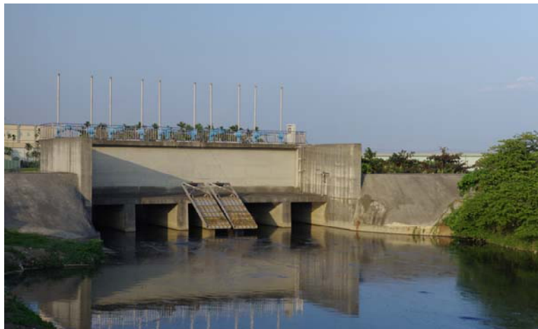
(b) Culvert system as part of an irrigation and flood control system on Tungkang River (Taiwan) on 27 December 2015
