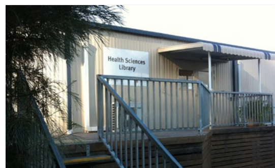
From top: Toowoomba Library, Bundaberg Library, Rockhampton Library
