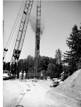
Figure 12 – Ground surface geophones on line with pile being driven
