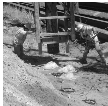
Figure 10 – Spotting pile and showing plastic bags containing cables from buried sensors
