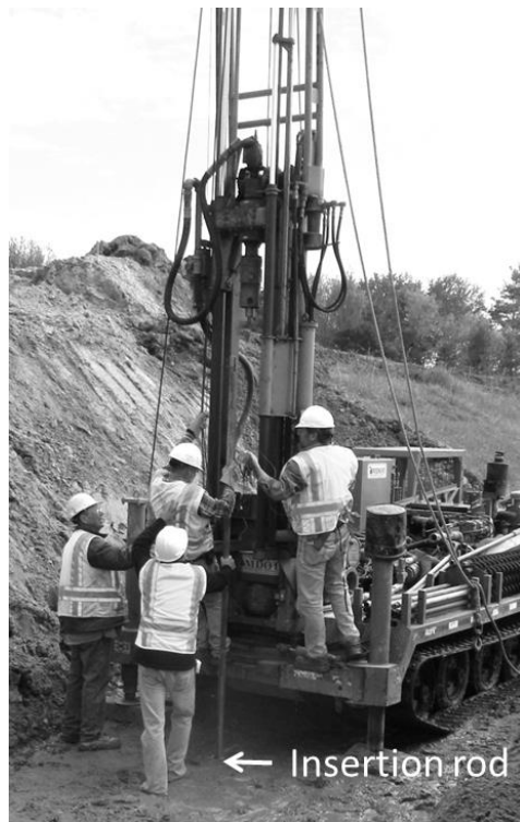
Figure 9 – All-terrain drill rig installing sensors using hydraulic thrust
