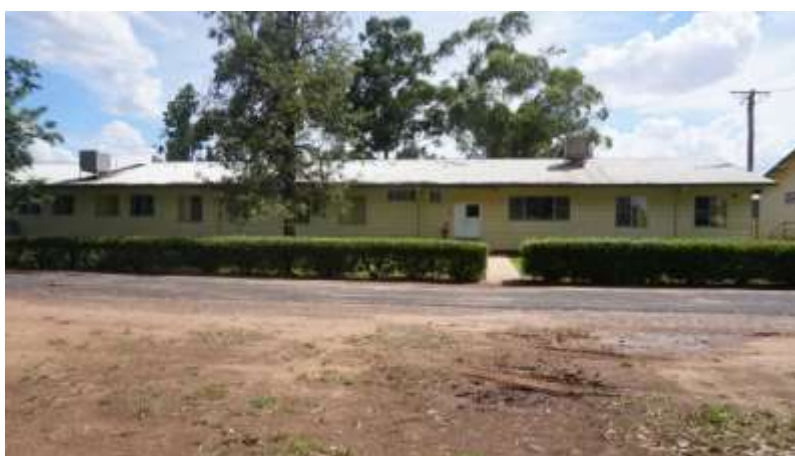
Figure 10.2. CSIRO Mitchell Laboratory at Trangie, 2016. The building is now part of the NSW Department of Agriculture research farm (photo Douglas Lawton).
