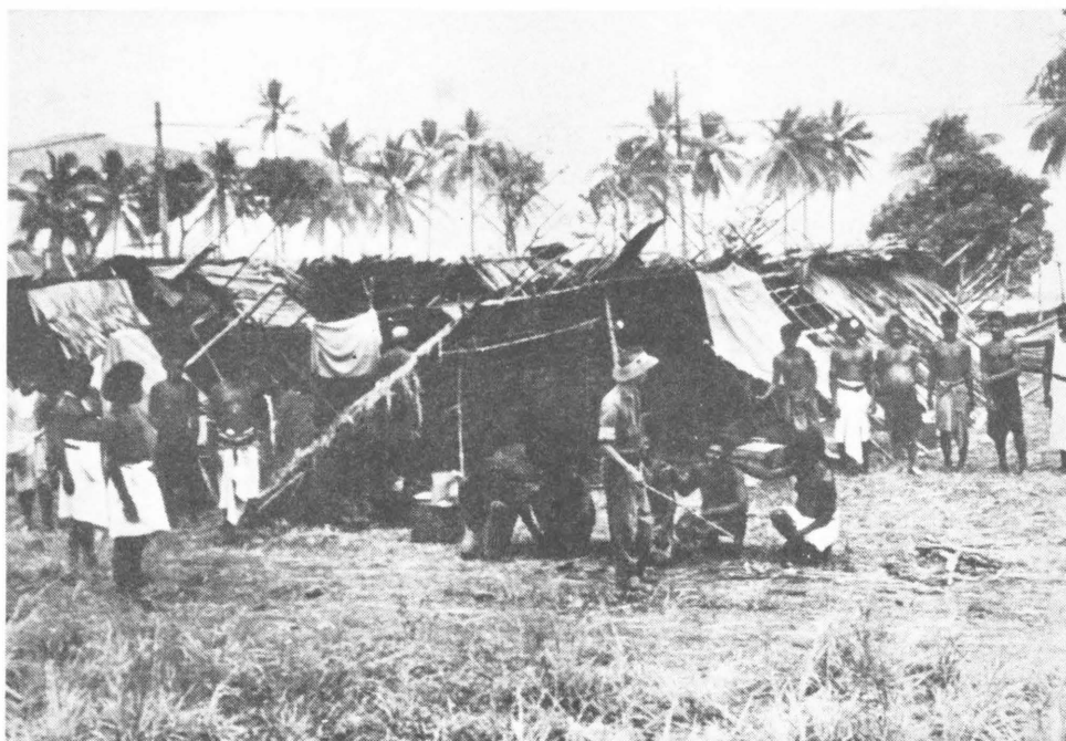
Plate 13. Within a few hours after a big fire had swept through the village of Hanuabada which housed 3000 labourers, the men had erected palm thatched lean-tos and were issued with tents. The labourers remained in a temporary village until other housing was provided.
