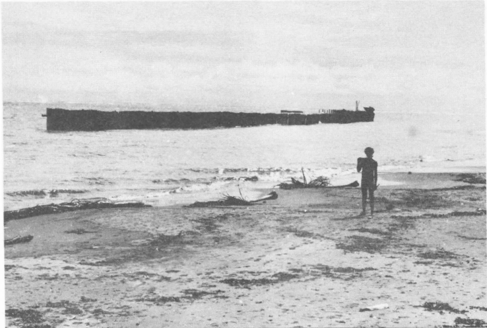
Plate 10. Long shot of groyne built by 2/4 Australian Field Squadron, Royal Australian Engineers, in order to divert the flow of the Lakekamu River. Mirivase, 7 September 1943.
