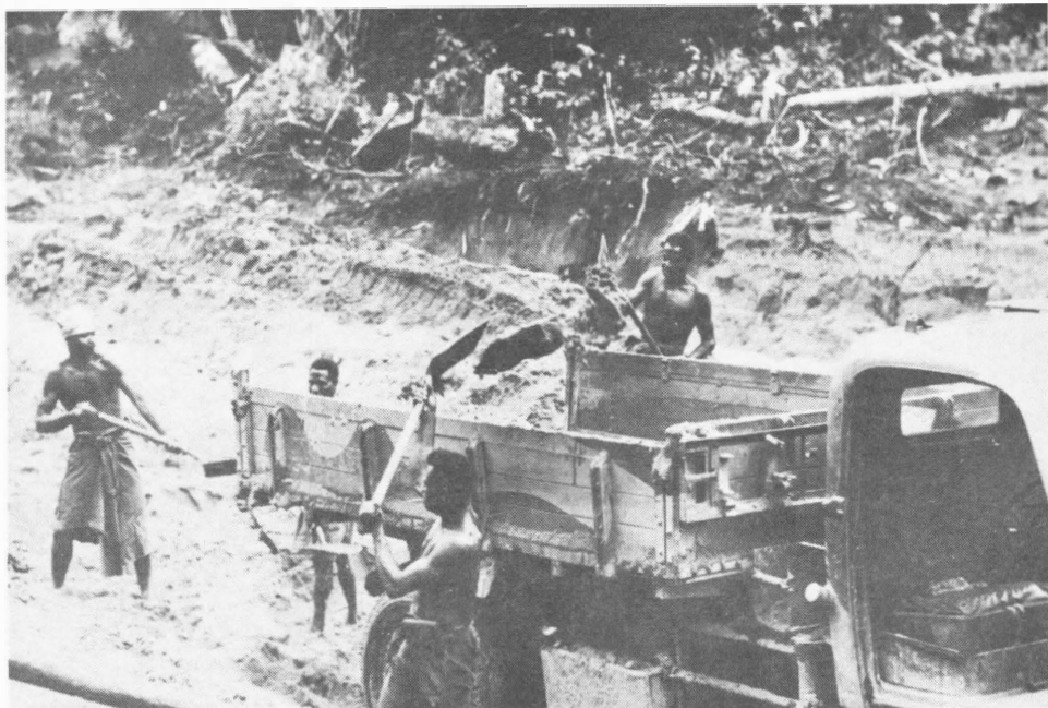
Plate 8. Labourers loading trucks with sand after bulldozers had cleared away overburden, Wau-Bulldog Road (later called the Reinhold Highway), New Guinea, 8 July 1943.
