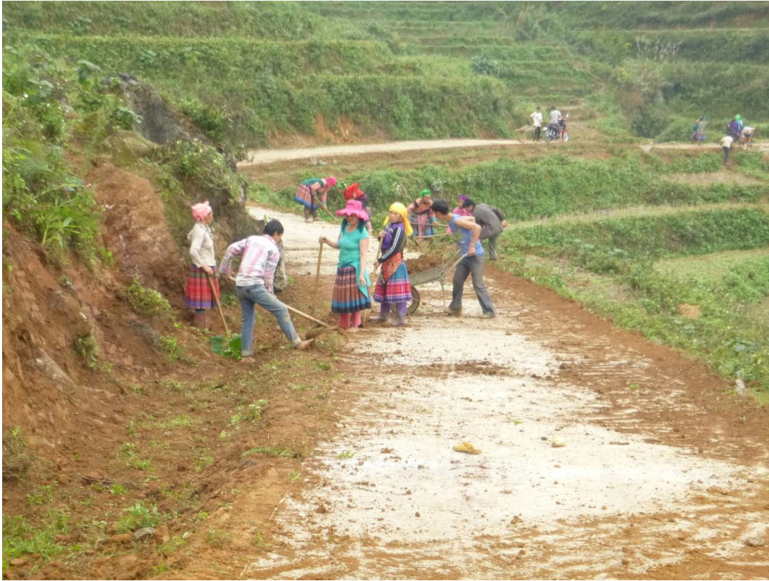
Photo 5.2: Villagers working on a rehabilitated commune road under the ‘New Rural’ programme of the government
