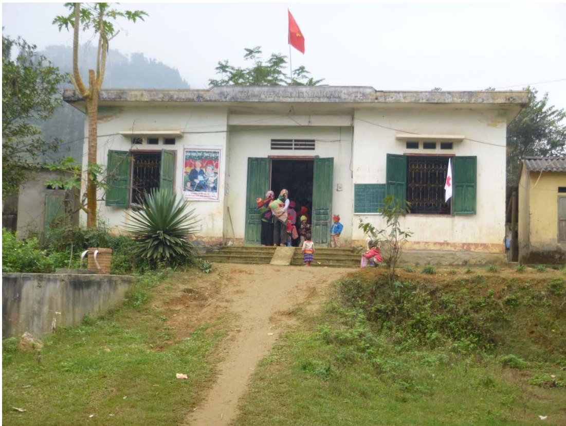
Photo 1.6: The commune health post in Vĩnh Thủy
