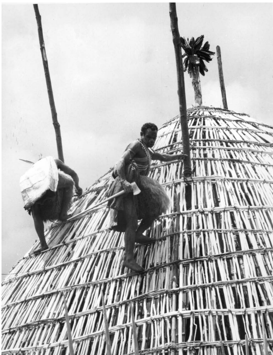
Figure 1 The building of the chimya ceremonial house
