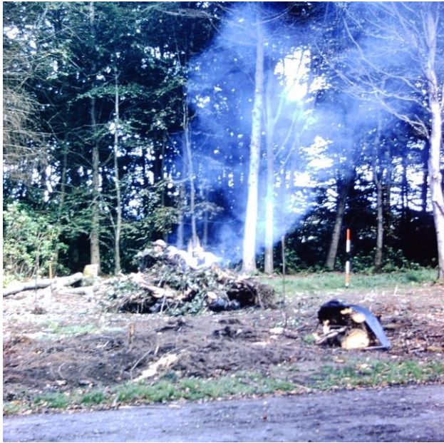
Figure 23. Clearing the North Side September (1952). AGT.
