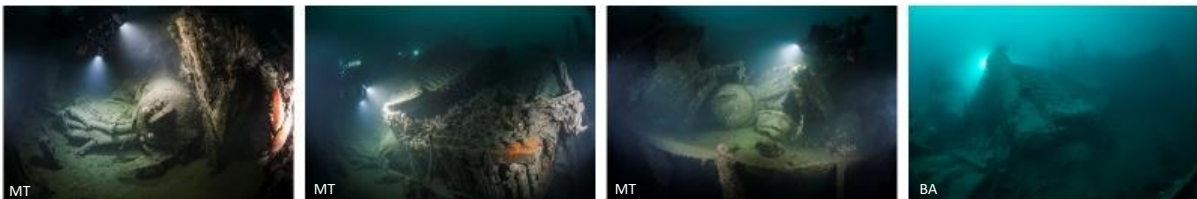
Figure 32: Babcock and Wilcox boilers
