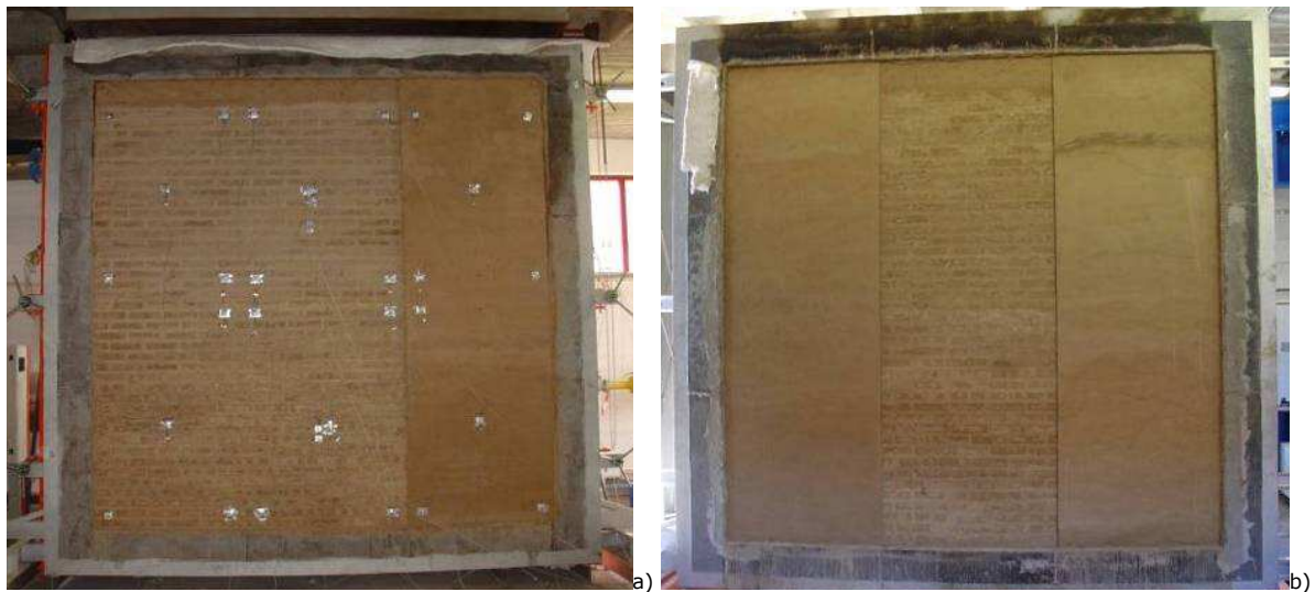
Fig. 1 a) External face and b) inner surface of the constructed wall, infilled in a reinforced concrete frame mounted to test for fire resistance at the LERF laboratory.
