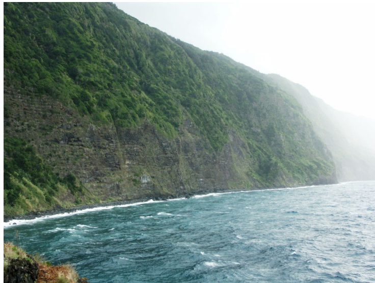
Fig. 3.11 – This picture was taken from Fajã das Almas looking southeast and shows a part of Rosais lava sequence forming the shore line behind Fajã das Almas. This lava sequence is located on the south shore of São Jorge and is formed by the pile up of relative thin lava flows.
