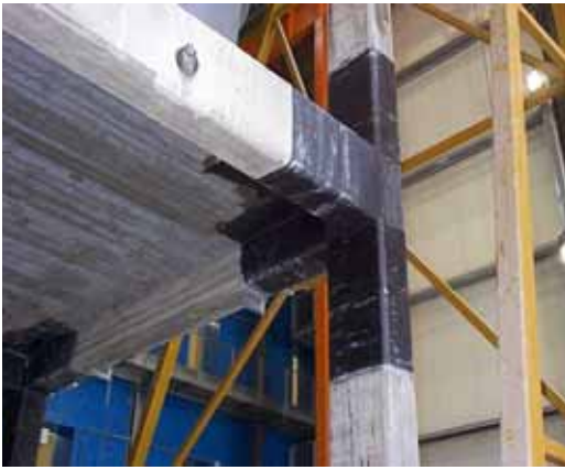
Figure 9. Member ends wrapped with CFRP
