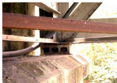
Figure 3: Fixed support in the north abutment [4].
