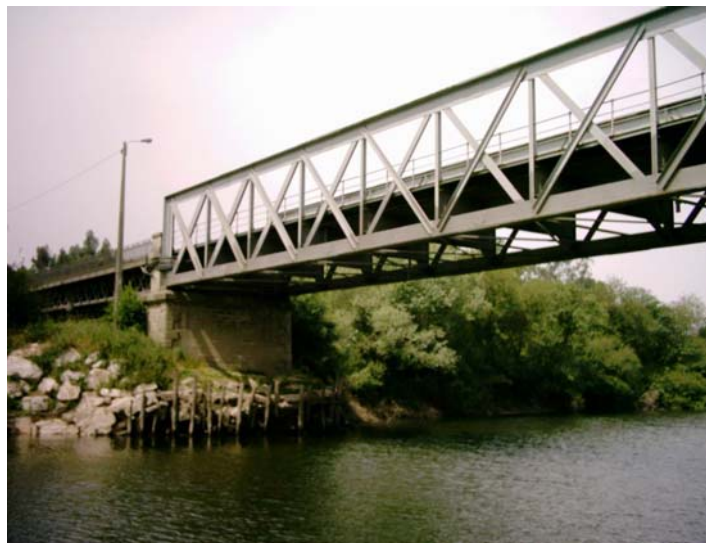
Figure 1: General view of the bridge S. João de Loure [4].
