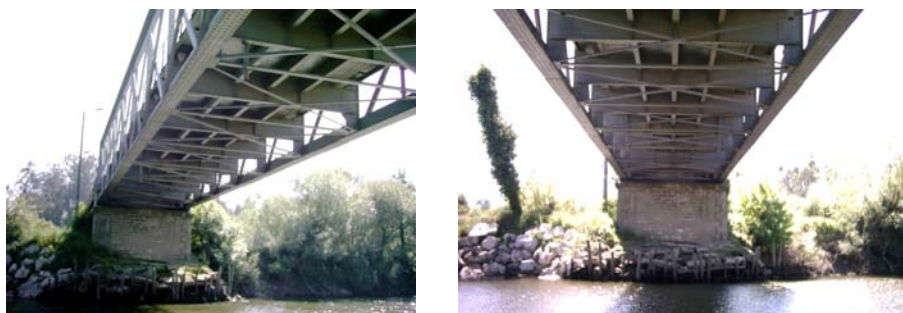
Figure 4: Inferior views of the bridge S. João de Loure – bracing system [4].
