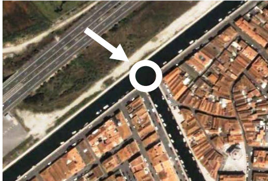
Figure 1 – Localization of the bridge
