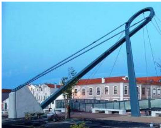
Figure 3 – Side view of tower, stay-strips and stay- cables
