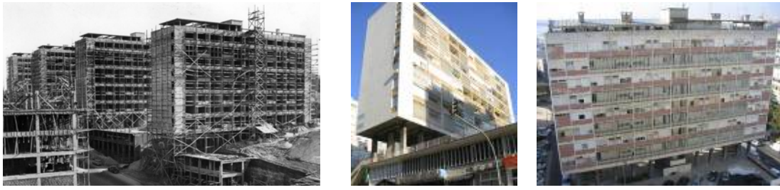
Figure 1. General views of the building block under analyses
