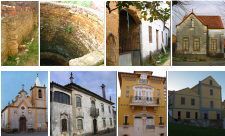
Figure 1: Examples of existing adobe constructions in Aveiro district.
