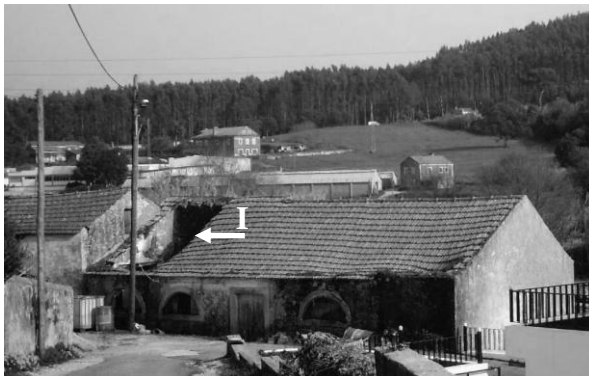
Figure 1. Watermill building's condition in 2000
