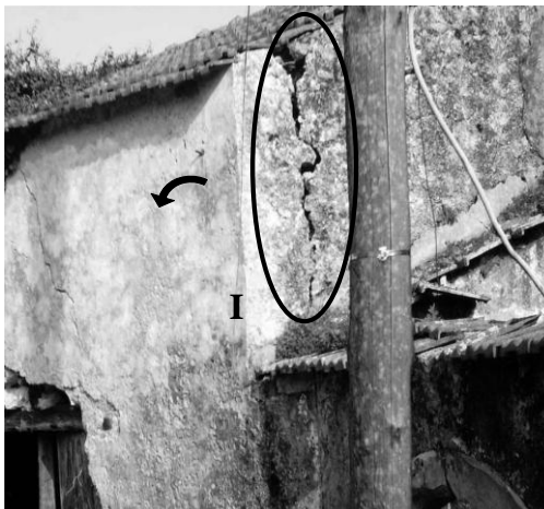
Figure 9. Vertical crack, 2007
