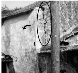
Fig. 6.2. Vertical crack, 2007
