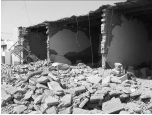
Figure 5. Out-of-plane failure.
