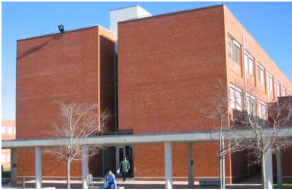
Figure 7. Photography of the characterized physics department building.
