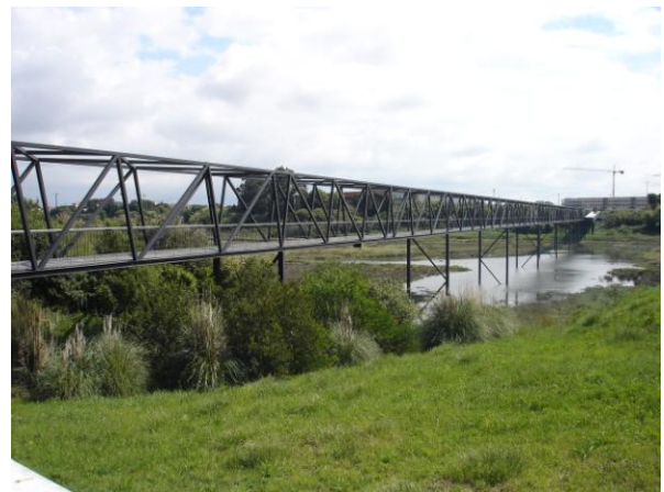
Figure 6. Photography of the characterized footbridge.
