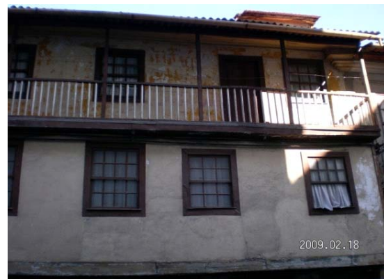
a) Exterior granite stone masonry walls
