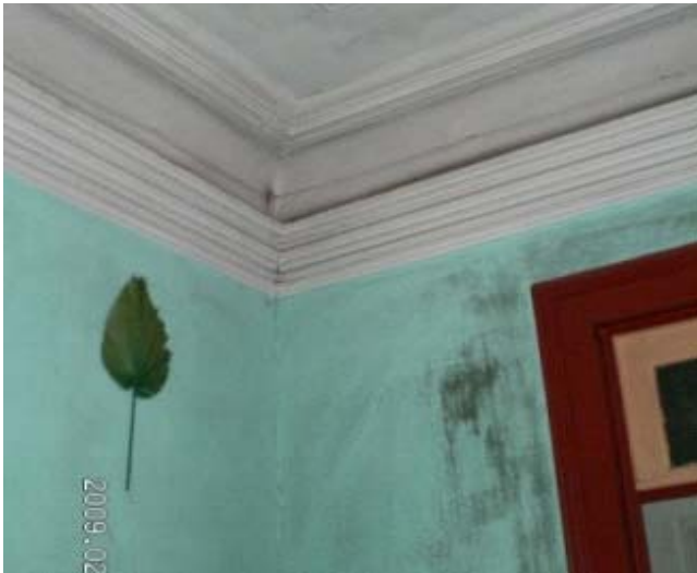
Fig.8 - Conservation state: Good conditions
