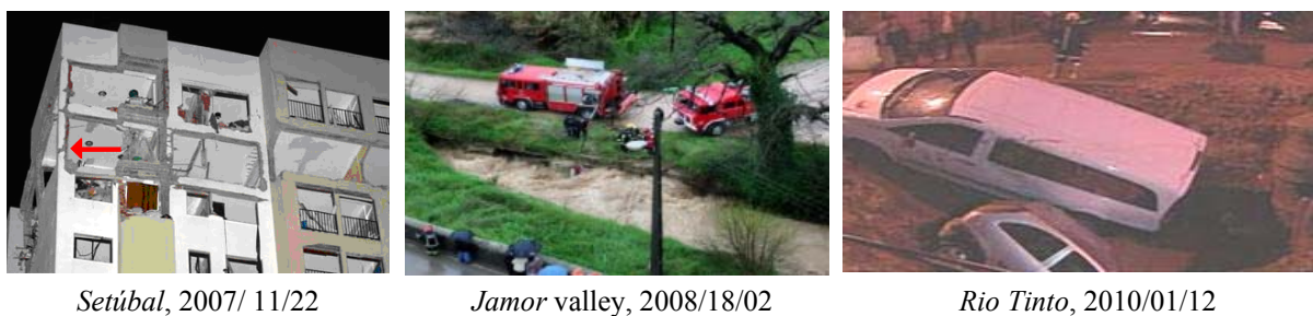
Fig. 1 Recent vulnerable failure scenarios occurred in Portugal
