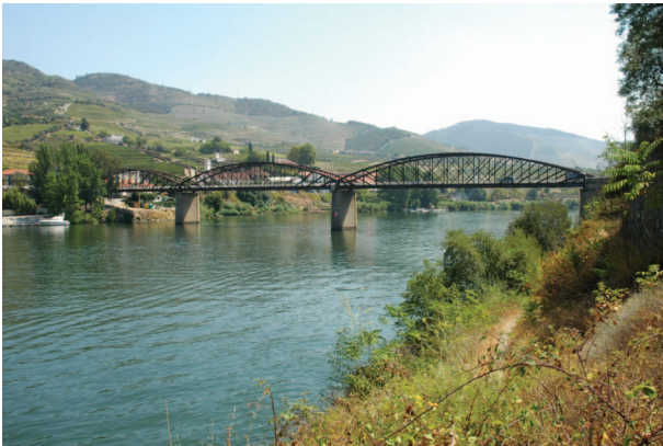
Figure 1. General view of the Pinhão Bridge.
