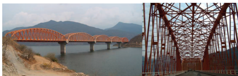
Figure 6. General view of the Infiernillo II Bridge.
