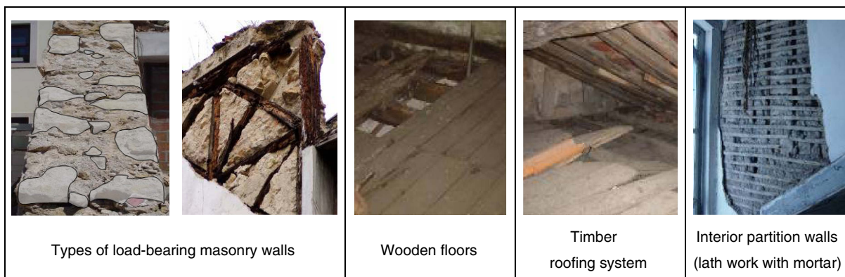
Fig. 3. Construction details of old housing
