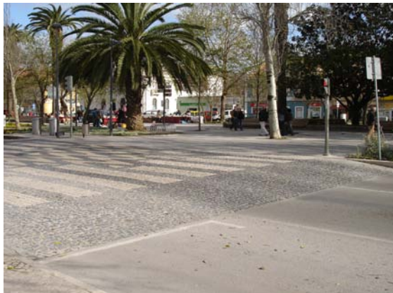
Figura 64 – Travessia pedonal elevada, Setúbal
