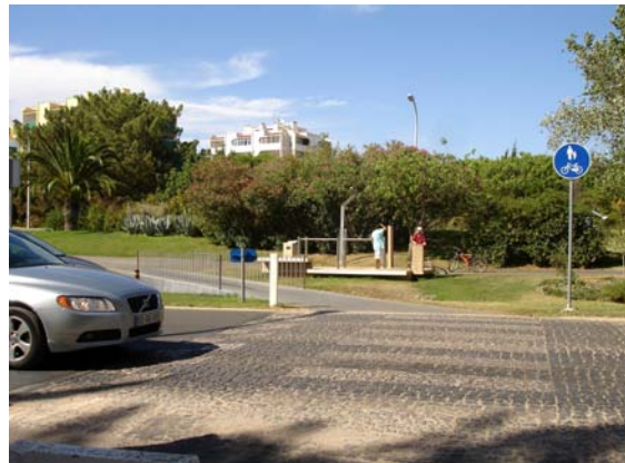
Figura 65 – Travessia pedonal elevada, Vilamoura (Loulé)
