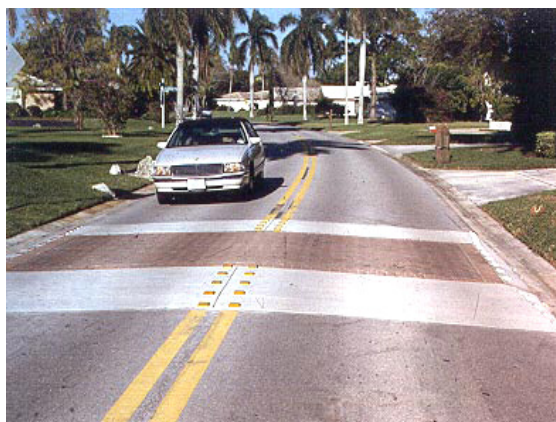
Figura 52 – Lomba trapezoidal (Ewing, 1999)
