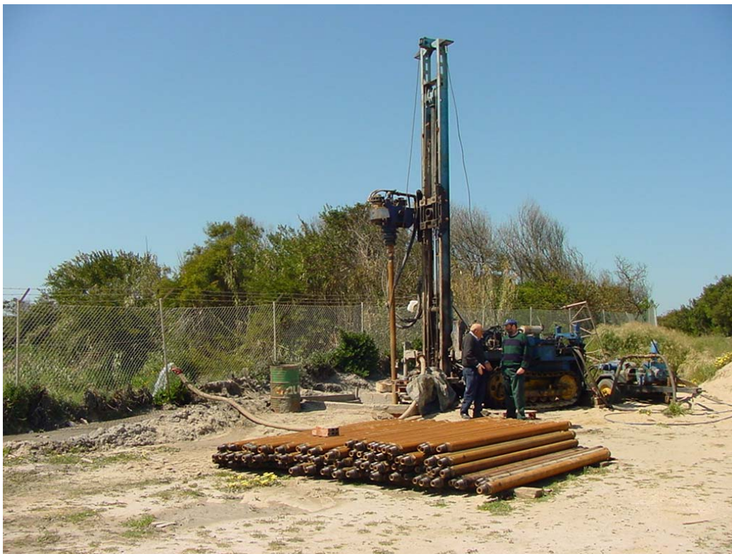
Fig. 1.4 Artesian borehole drilled in April 2002 in the Aveiro Cretaceous aquifer at the Areão beach (south of Vagueira).
