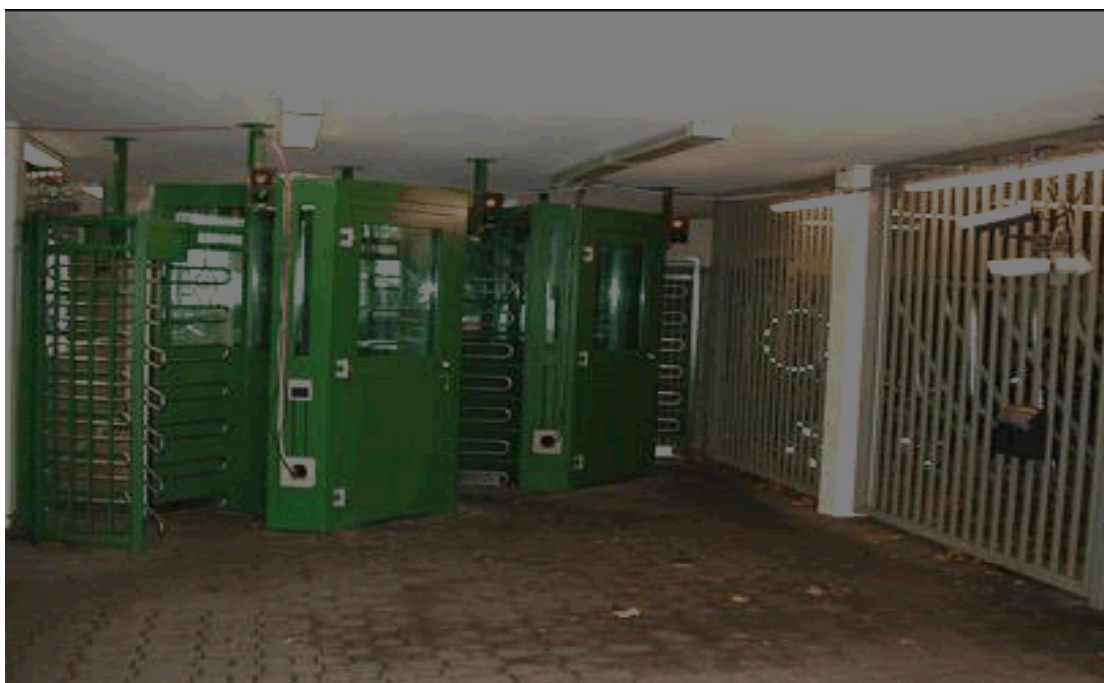
Figure 15: The entrance where the system evaluation was conducted 50
