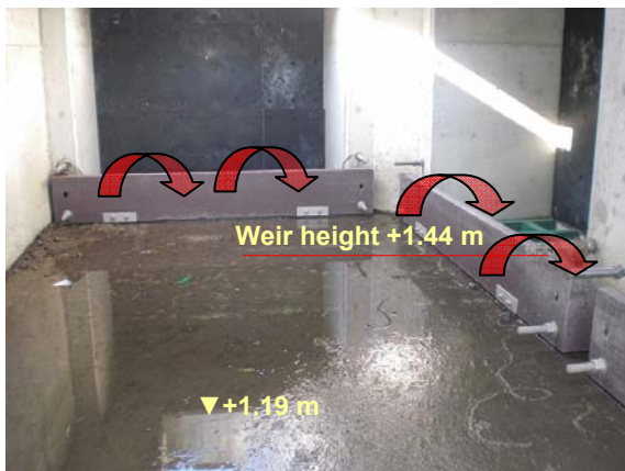
Photo 3-3 Overflow Weir (taken from ③)
