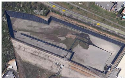
Figure 1. Django Reinhardt retention / detention basin (source : Google map - 2012)
