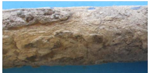
Wood firing power plant No Thermal cycling + 520 °C
