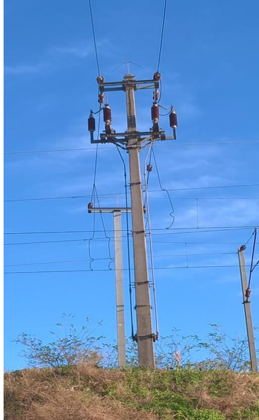
Figure 36: Post of North Line
