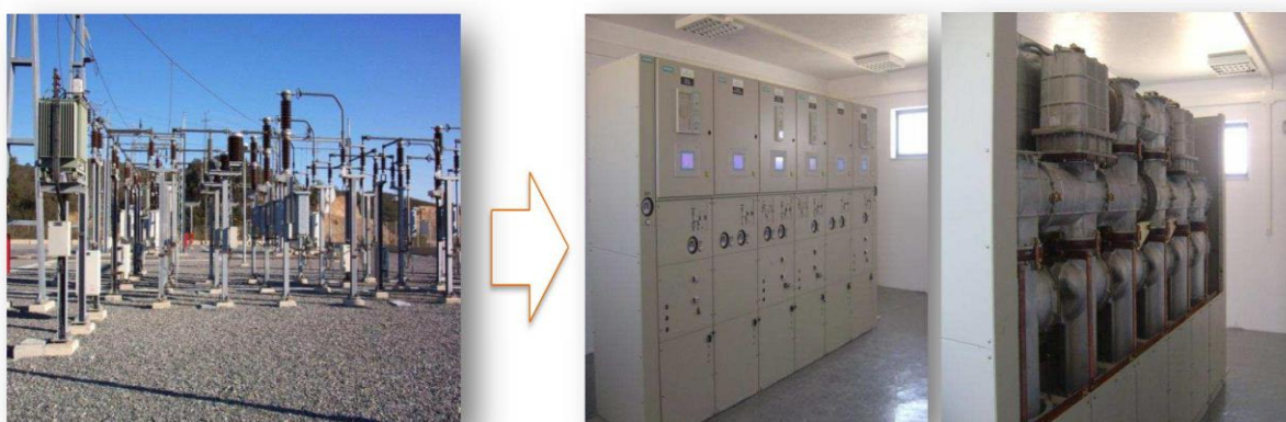
Figure 28: Comparison between traditional and new GIS substation
