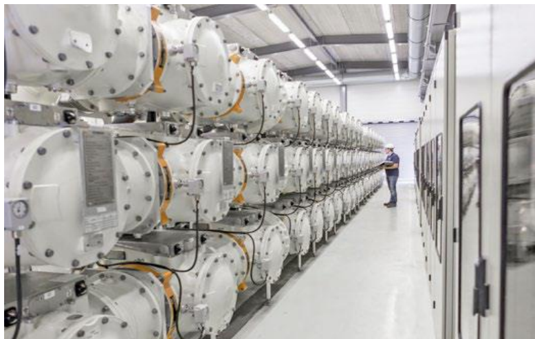
Figure 27: 8DN8 GIS for a rated voltage of 110 kV
