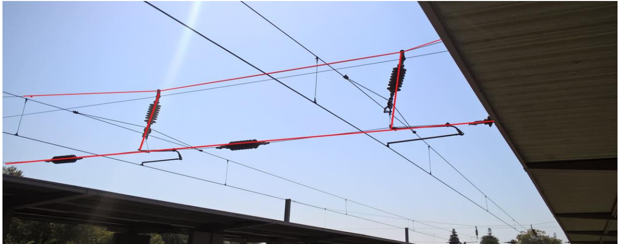
Figure 41: Flexible Portics at Rua do Jau:
