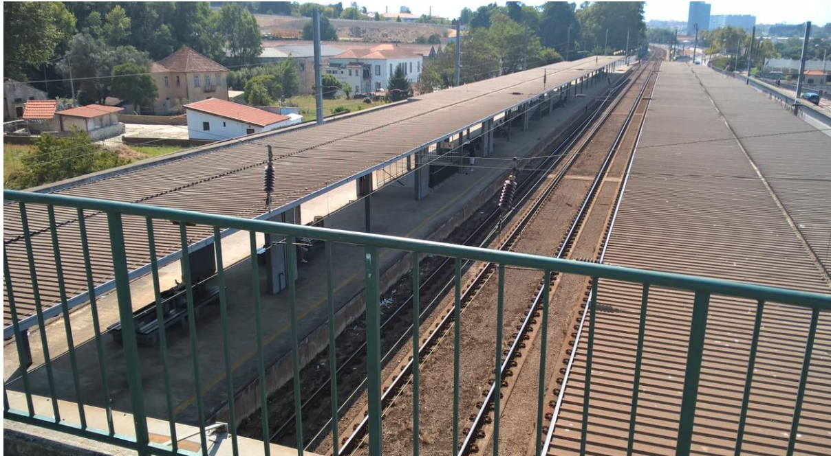
Figure 39: Rua do Jau station
