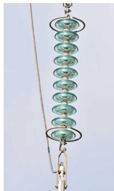
Figure 5: Airline flexible insulator | Material: Glass
