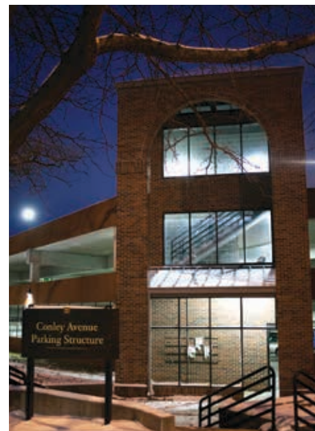
The Conley Avenue Parking Garage before (top) and after the installation of LED lights.
