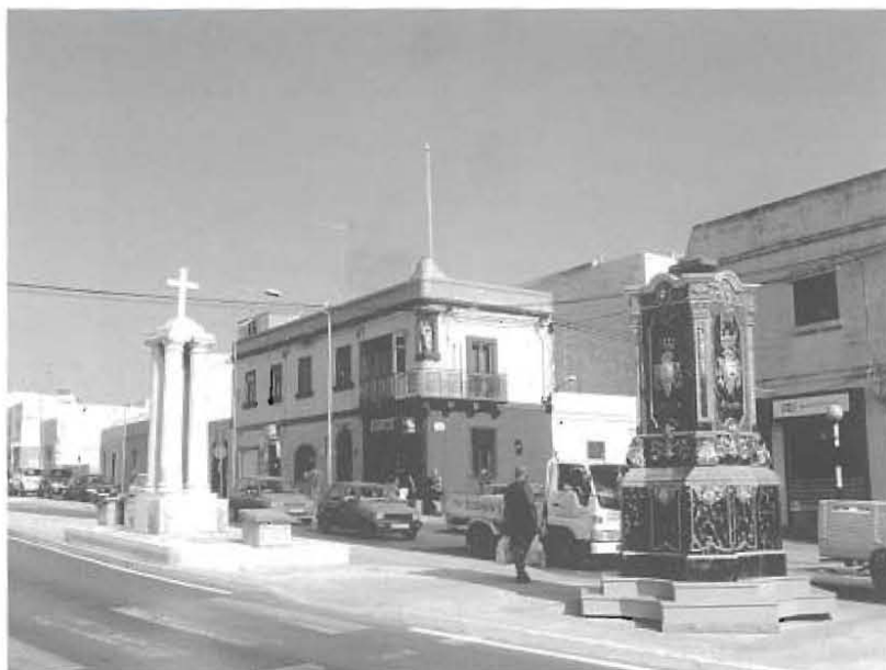
Fig.1- The road junction where the four principal streets in il-Fgura met. In this area was situated the old church, whilst the entrance to Carmel Street is visible to the right of the picture.
