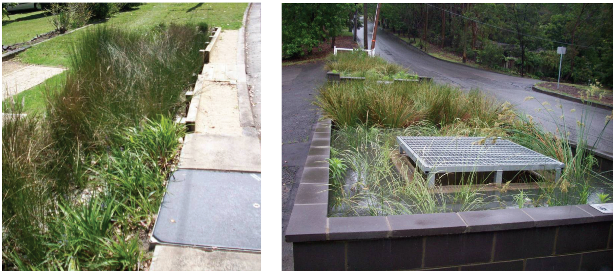
Figure 1. Biofiltration system at Kooloona Crescent, West Pymble (Left), and at Nimbrin Street, Turrumurra (Right)
