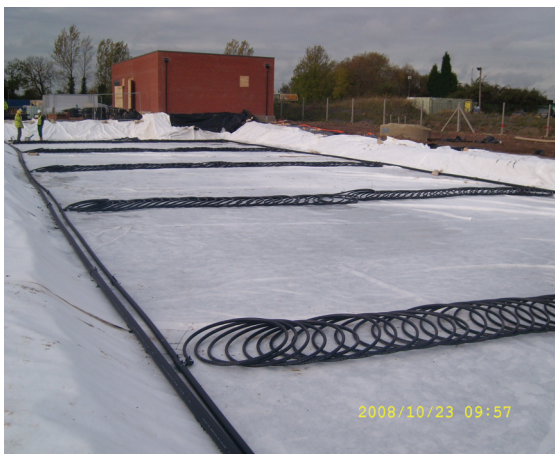
Figure 2. A: site excavation and ground preparation, B: installation of the heat welded impermeable membrane, C: The GSHP collector loops, D: The completed paving surface.
