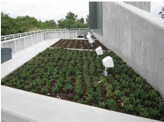
Figure 1 – Frontier Project Green Roof
