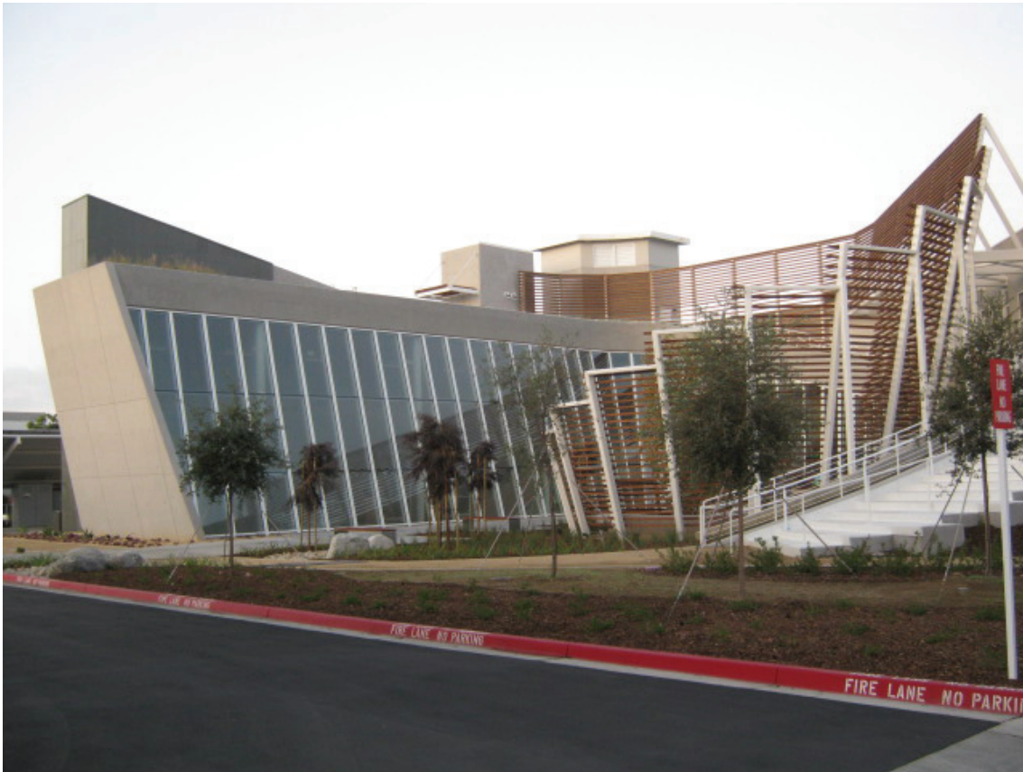
Figure 12 – Completed Frontier Project
