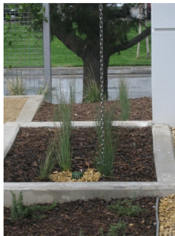
Figure 8 – Rain Chain and Capture Structure
