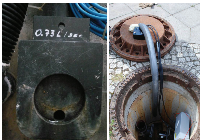
Fig.7: Conventional static and managed throttle
