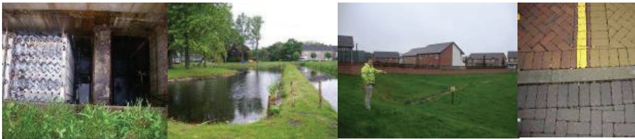
Figure 6 SUDS: lamella filter (Netherlands), sedimentation basin (Netherlands), swale (Scotland), pervious pavement (Scotland),
