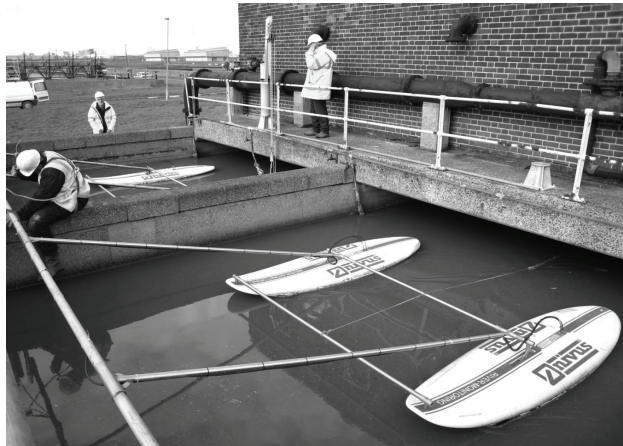
Figure 9: Float system using surfboards
