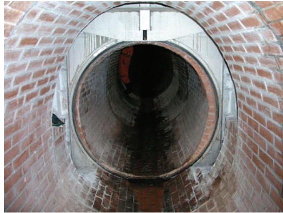
Type of flood protection closure in the sewer network in the City of Prague.
