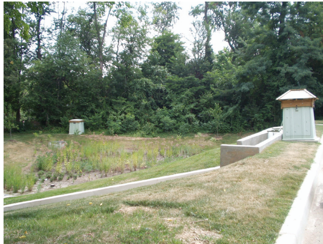
Figure 2. Silver Spring, MD bioretention facility.
