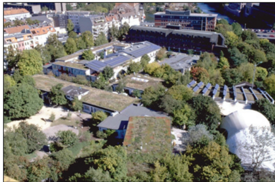
Figure 1 Extensively greened roofs in combination with 53 kW photovoltaic production (Schmidt, 2004)
