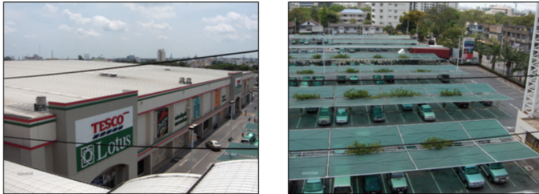
Figure 5 A roof of a shopping mall and its parking lots in Bangkok
