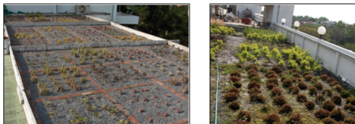
Figure 6 Green roof experimental plots at Mahasarakarm University, Thailand
