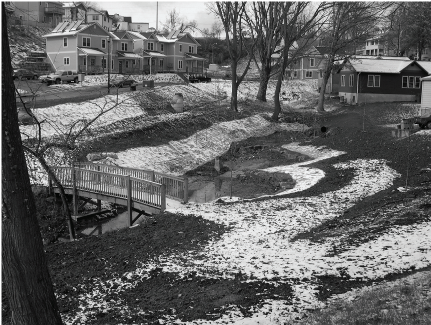
Under Construction (Photo Credit: Jon Calabria)
