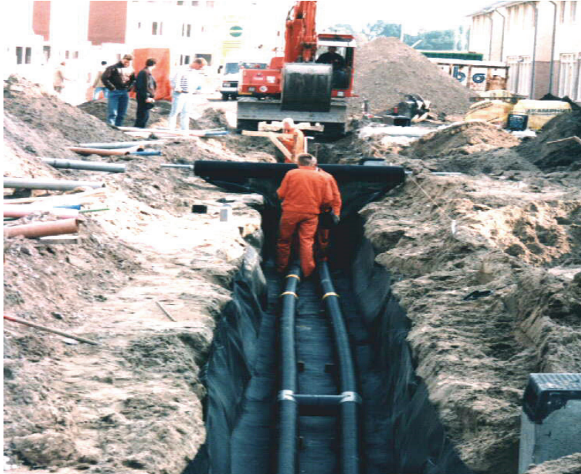
Construction of infiltration trench at Schellerhoek, Zwolle, Netherlands
