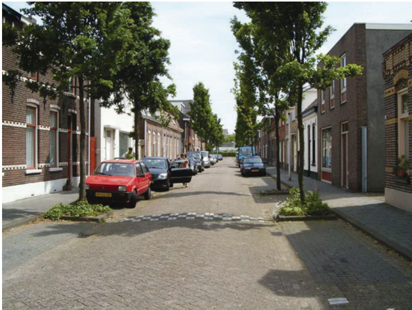
Run-off in the Runstraat in Eindhoven is disconnected to soakaways
