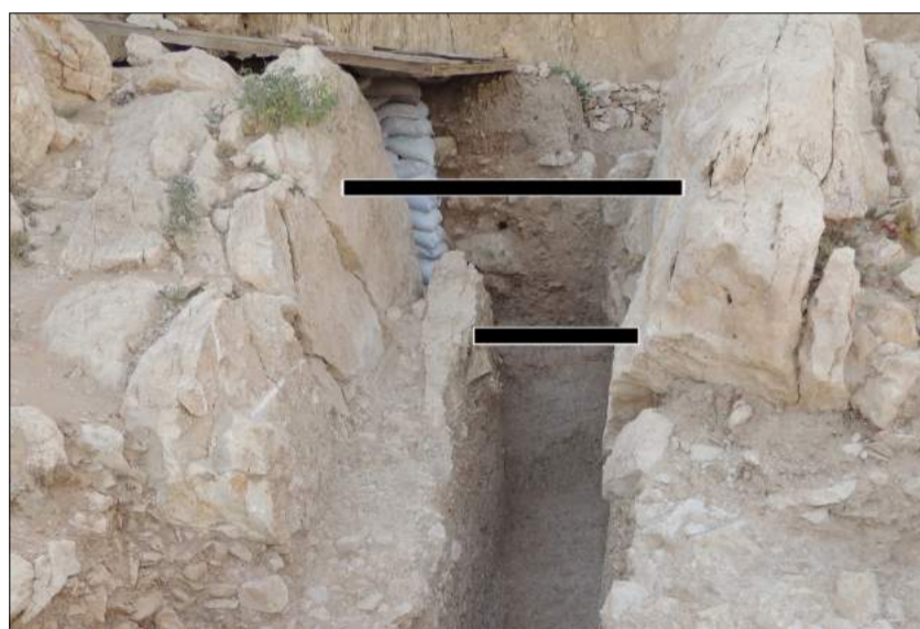
Fig. 7. Potential location of two floor props to prevent the blocks from falling into trench 38.
