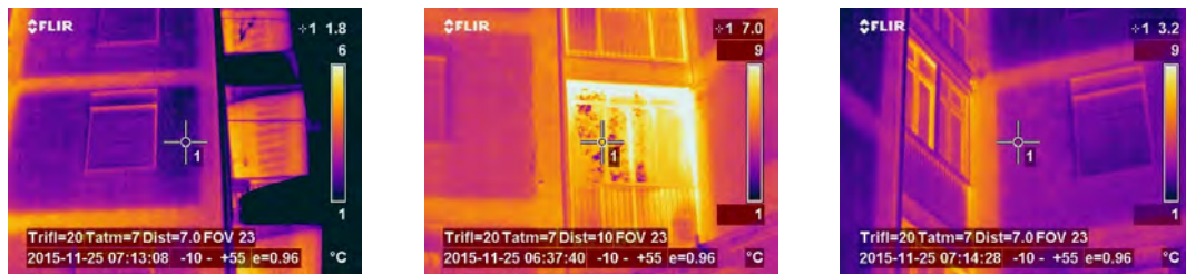
Figure 6. Thermal bridge detection with on-site thermography.
