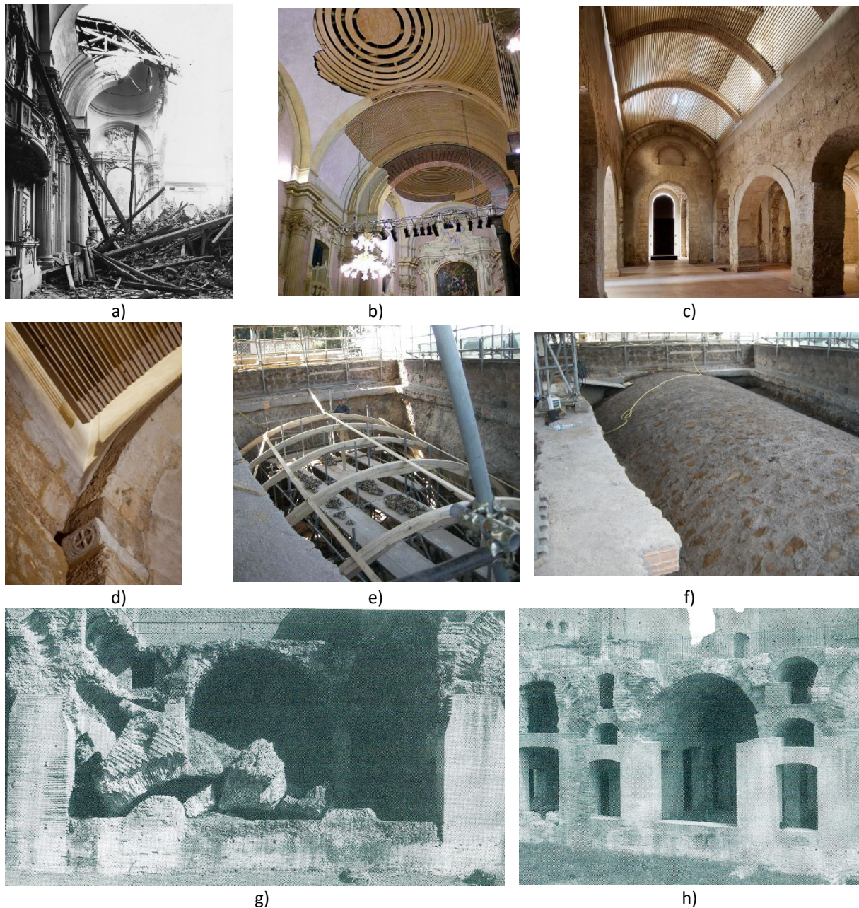
Figure 1: Examples of either partial or complete reconstruction: San Filippo Neri Oratory in the city of Bologna a) soon after the 1944 bombing and b) after restoration of 2000; c,d) San Peter's Basilica in Siracusa; e,f) Domus Tiberiana in Rome; g,h) huge vault of Villa Adriana Stadium in Tivoli .
