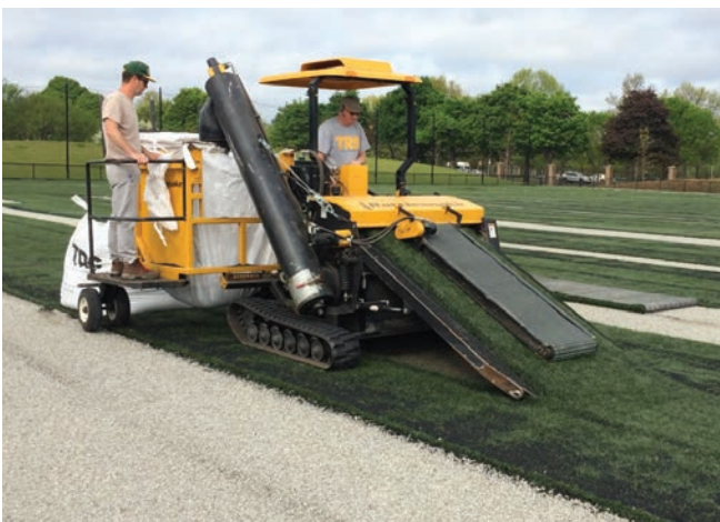
Removal of turf taking place
